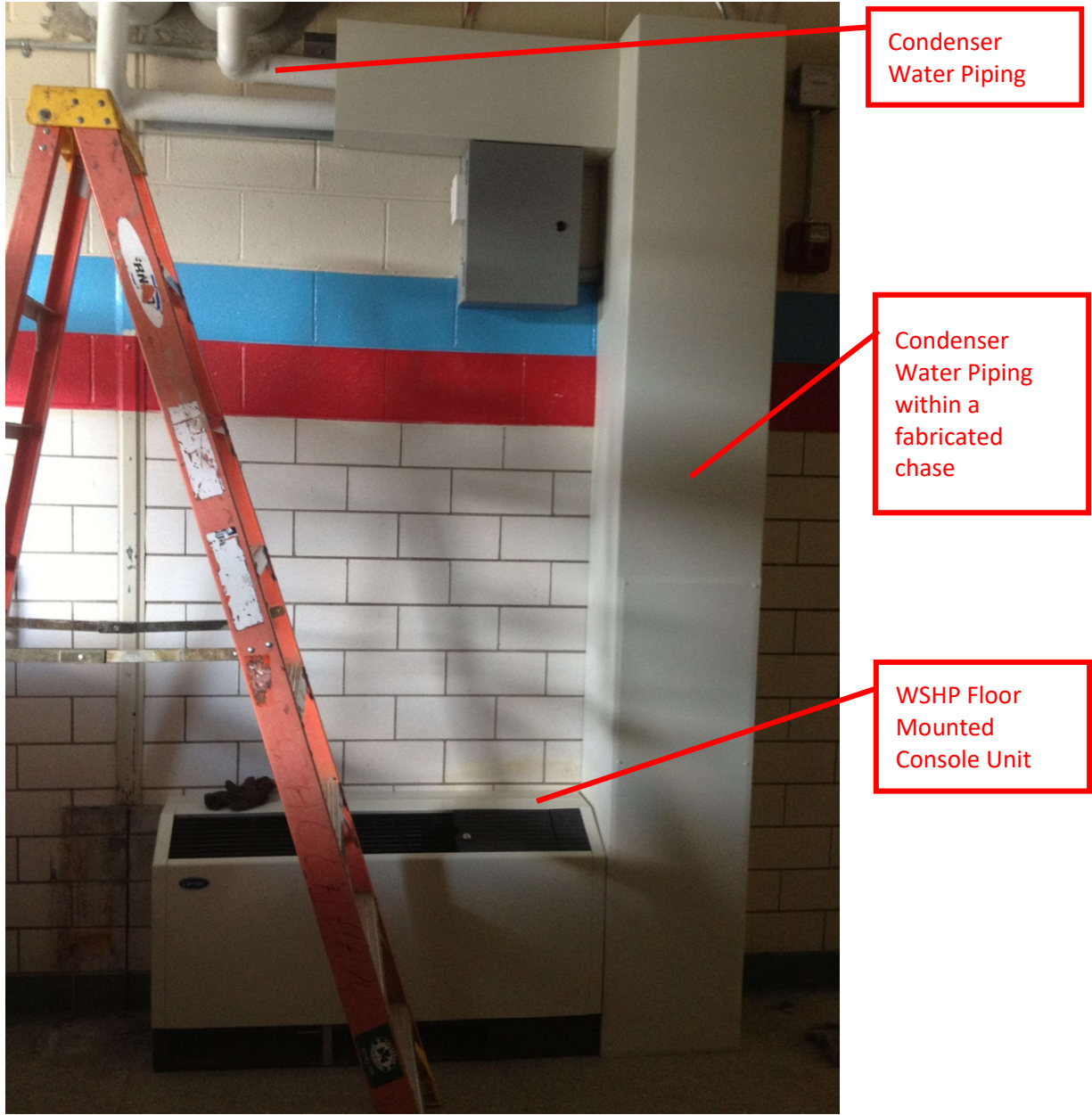
WSHP Floor Mounted Console Unit Installation Example
